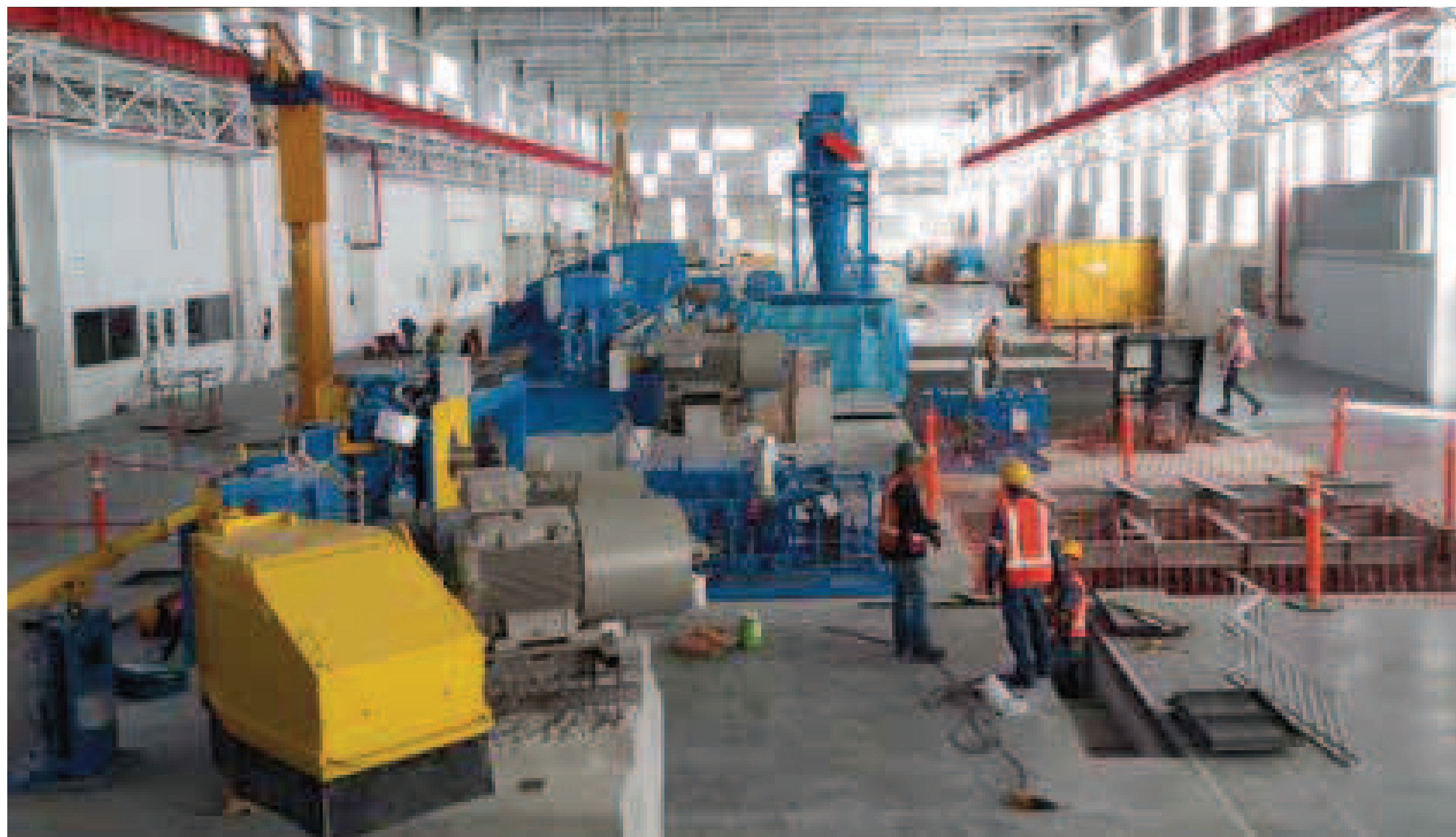
...during the installation of Aluminium Rod Mill 5 tph.
