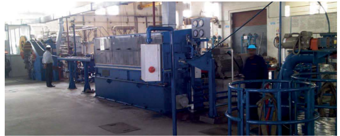
Continuous-Properzi Zinc line.
