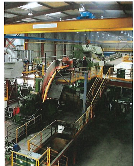
Typical Properzi CCR CU Line
