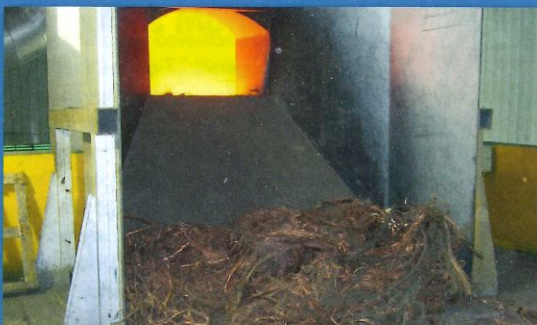
Properzi Vert-Ref Furnace loaded with scrap with a minimum copper content around 93%.
