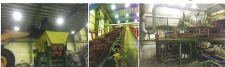
Loading of scrap into the refining furnace.
