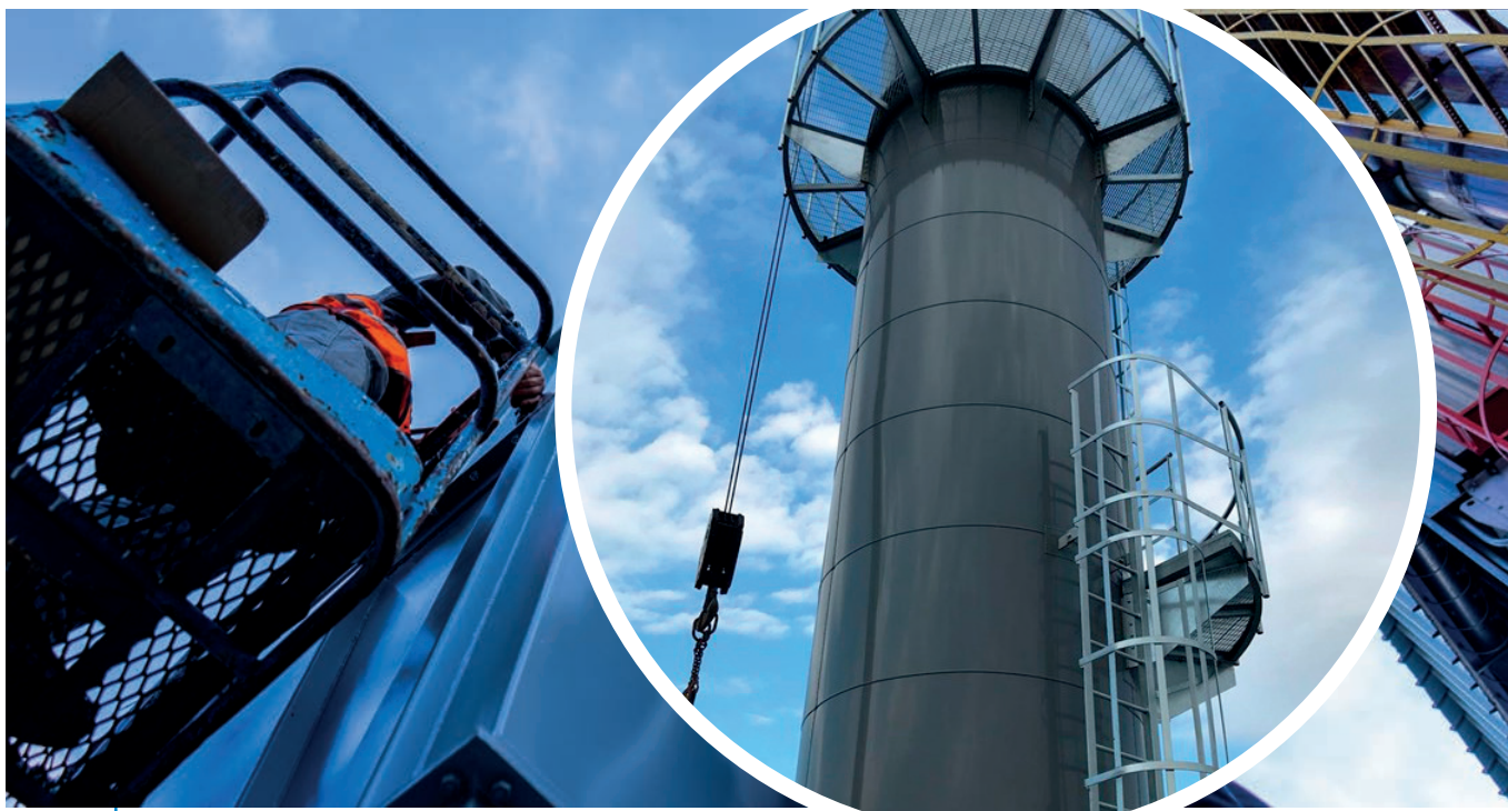
During Installation of a Fumes Treatment System
